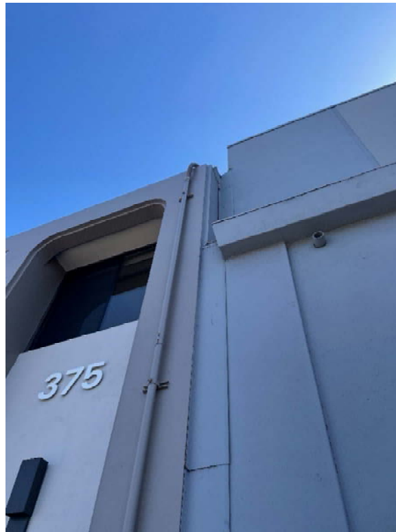
Image 8: Seismic Gap
