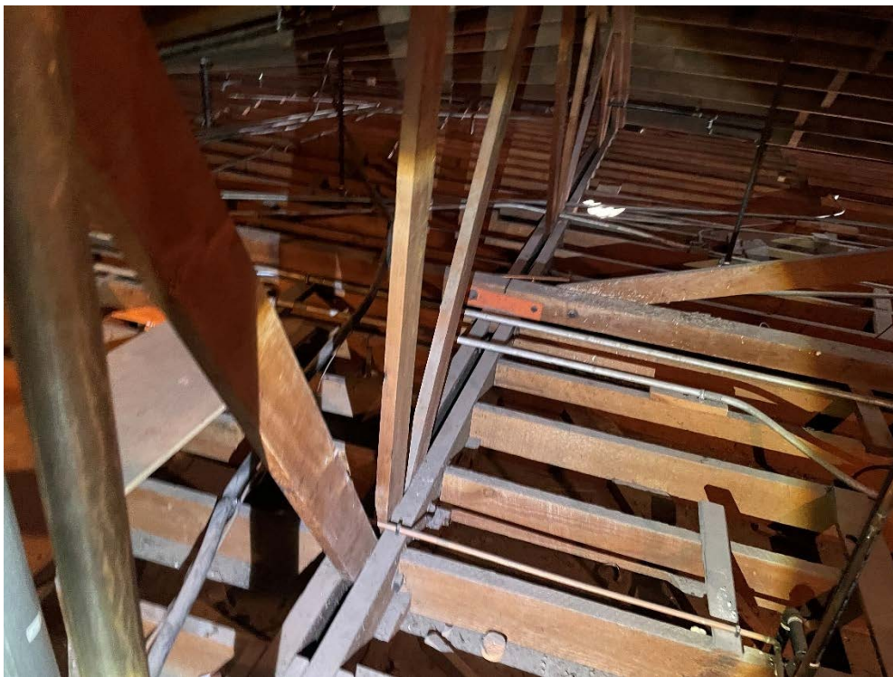
Image 4: Bowstring Roof Trusses
