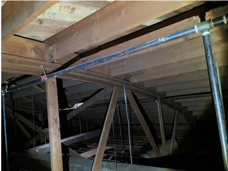
Image 3: Bowstring Roof Trusses
