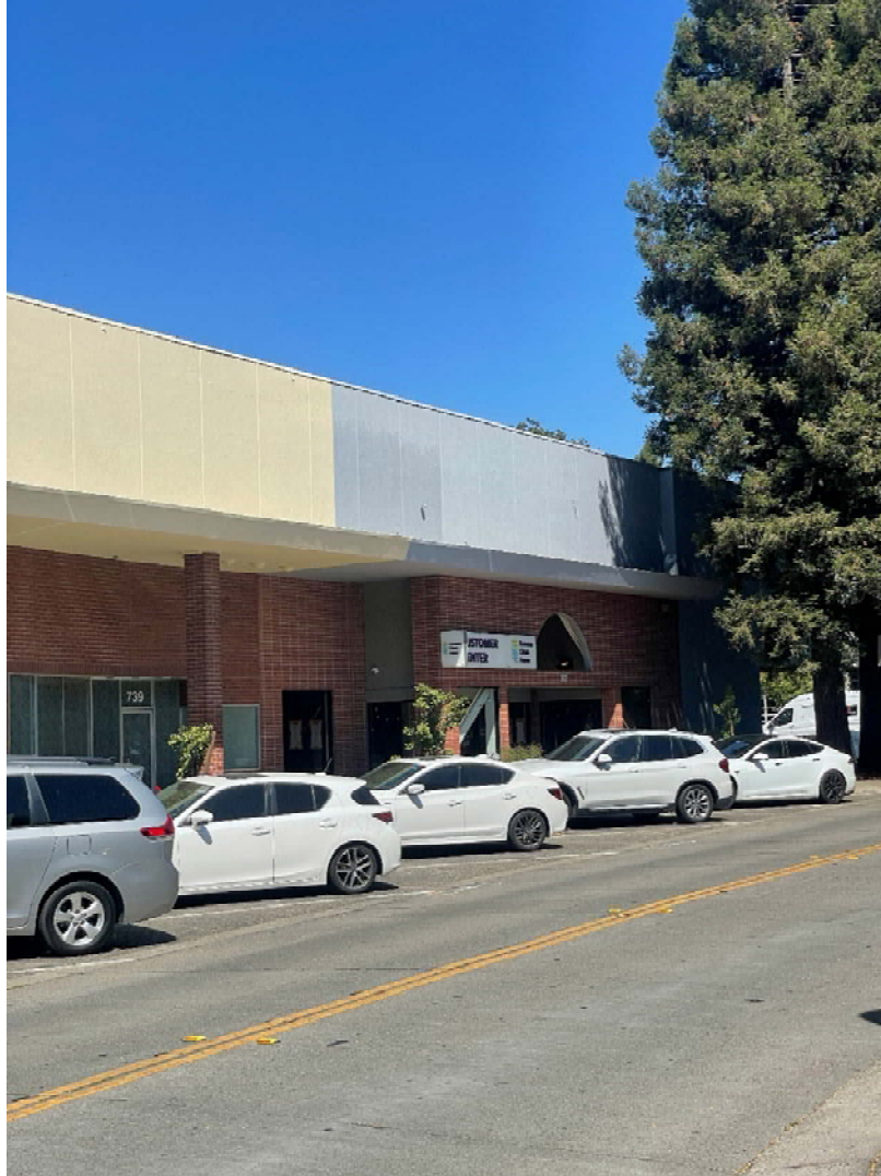
Image 6: North Elevation and Entry Brace Frame
