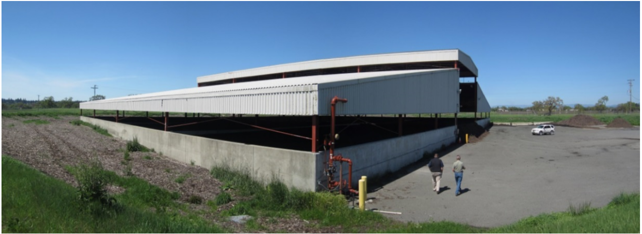
Figure 2-7: Alpha Farm Biosolids Storage Building
