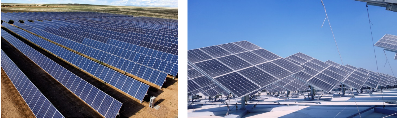
Figure B-2: Single-Axis and Dual-Axis Tracking Systems
