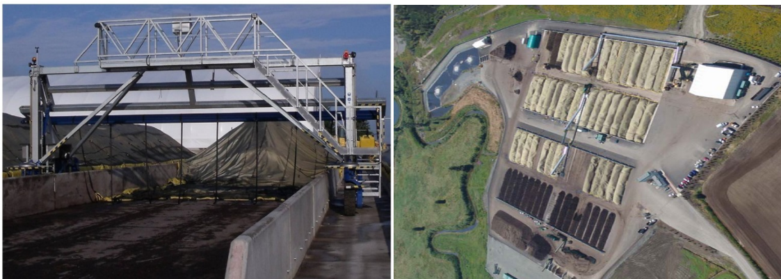
Figure 6-3 Covered Aerated Static Pile (CASP) Composting
