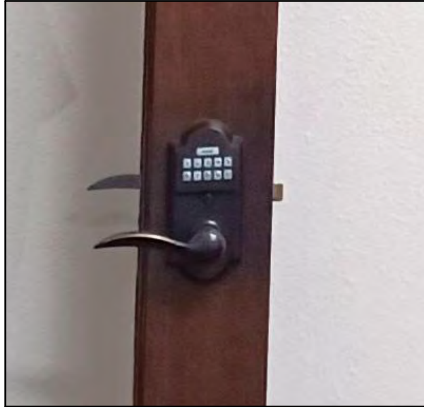
KEYPAD - LEVER - LATCH HARDWARE - TO BE REMOVED AND REPLACED WITH OWNER'S NEW STOCK LEVER/LATCH HARDWARE
