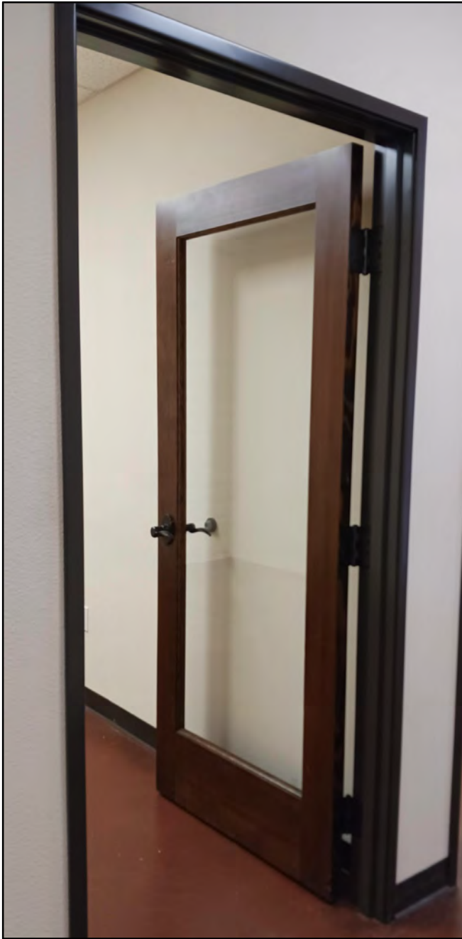
TYPICAL - LEVER - LATCH HARDWARE - (3) HINGE ON HOLLOW METAL FRAME - HINGE SETS TO BE REINSTALLED ON NEW DOORS. SEE SCHEDULE
