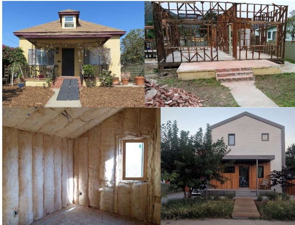
Figure 31: The Perlita Passive House: the original house was stripped to the studs, re-insulated, tested and made into an LA modern masterpiece of efficiency. 76
