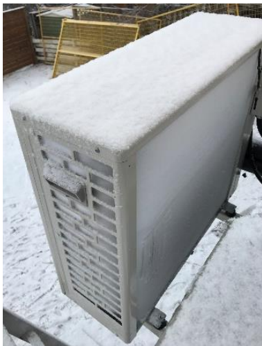
Figure 42: The Eco2 heat pump water heater compressor working outside in 5°F (-15°C) weather. 91
