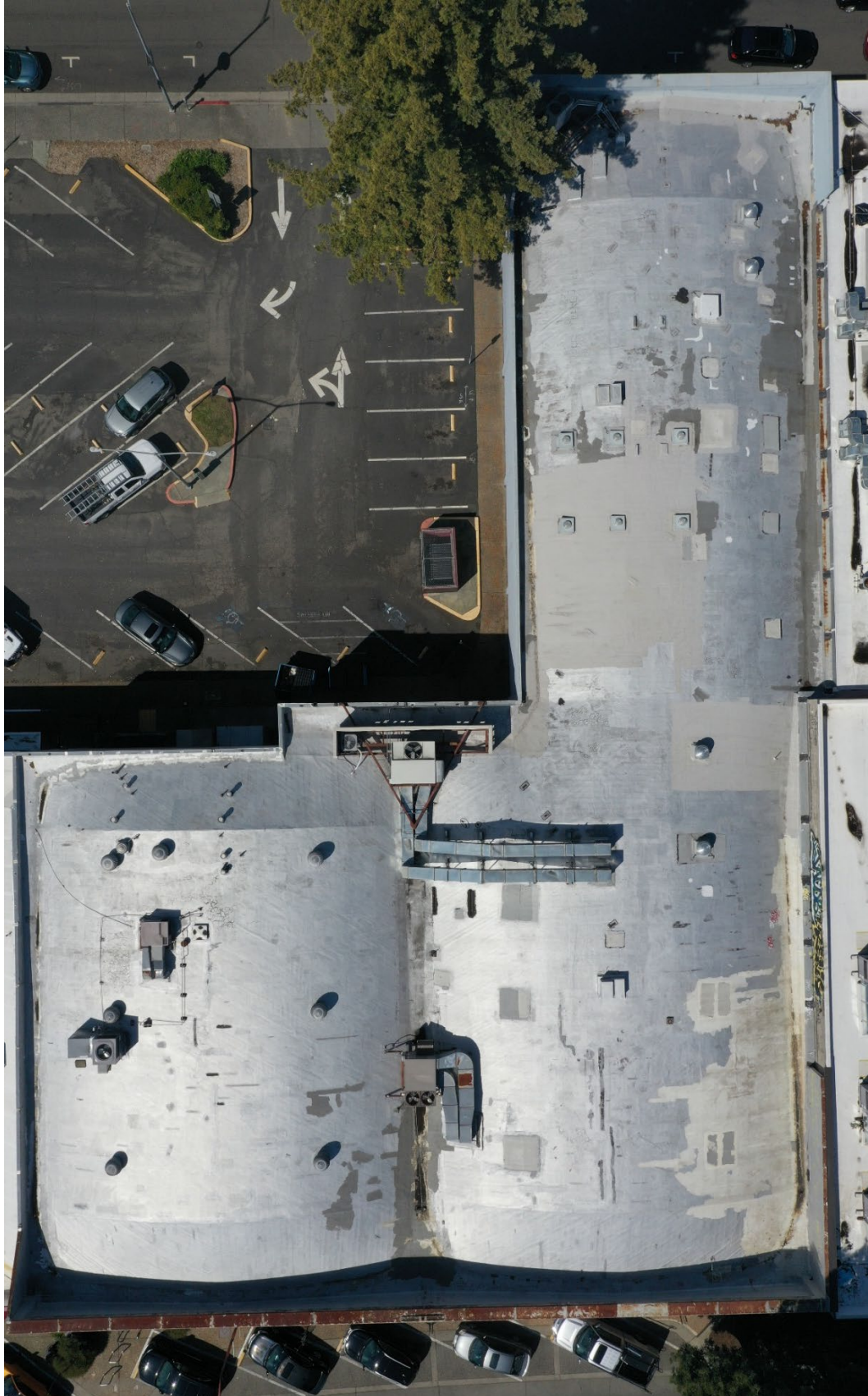
4 TH STREET ROOF OVERLAY
