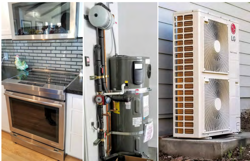
Figure 7 High efficiency induction cooktop, grid interactive heat pump water heater, and mini-split HVAC system 6
