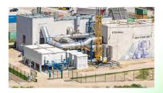
Stores thermal energy by using electricity to raise the temperature or changing the phase of a material. Discharged using a heat cycle that drives a turbine. Low round-trip efficiency due to heat cycle, but scalable to longer-durations due to lower material costs.
