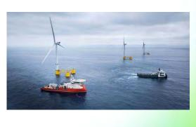
Floating turbines are placed on buoyant platforms tethered to the ocean floor with mooring lines. Suited for deeper waters—offers flexibility in site selection but involves more complex engineering.
