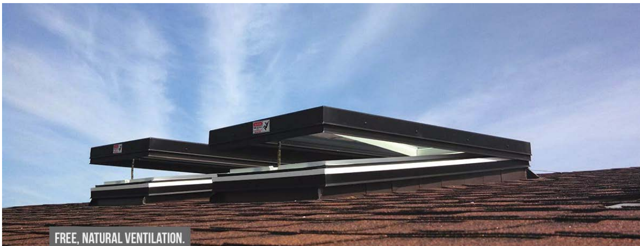
Figure 20. Example of venting skylight
