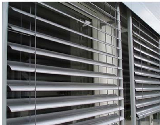
Figure 14. Example of motorized exterior Venetian blinds
