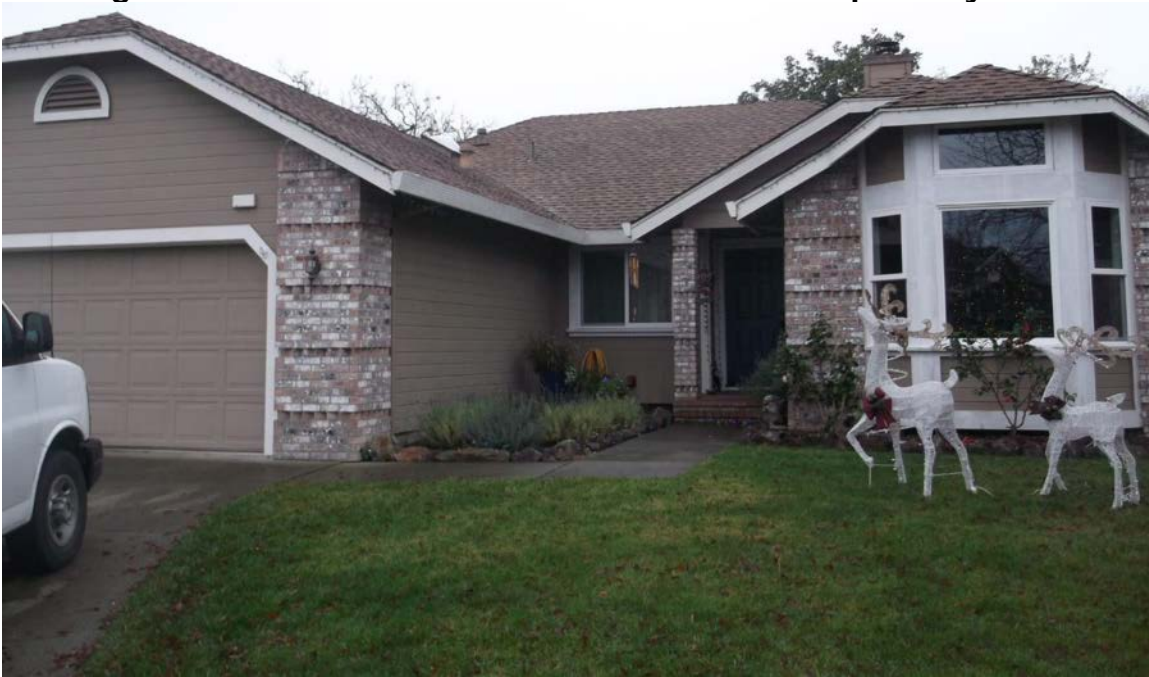
Figure 10 - Selected home to install the radiant panel system.
