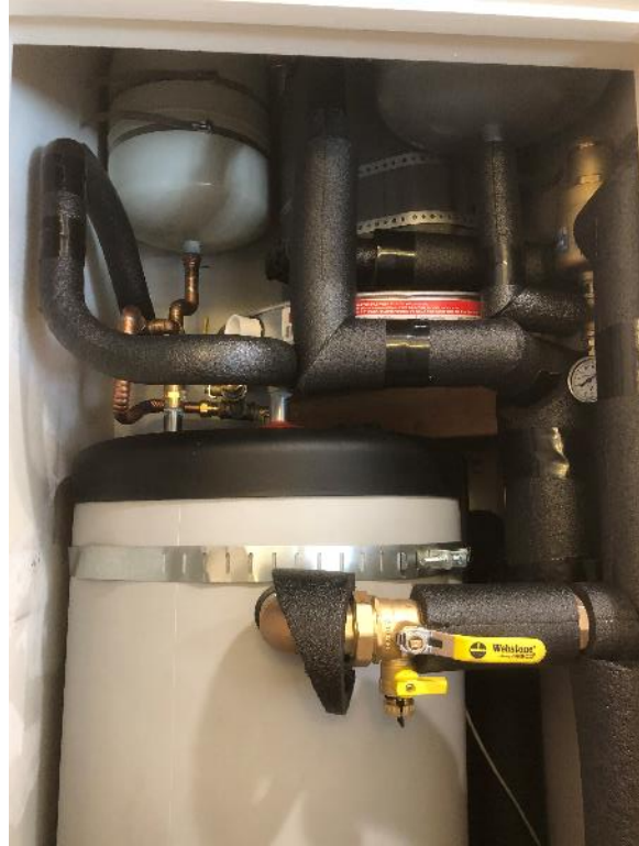
Figure 29 - Installation site of AWHP (left). Closet in laundry room holds indirect water heating tank, expansion, and backup tanks (right).
