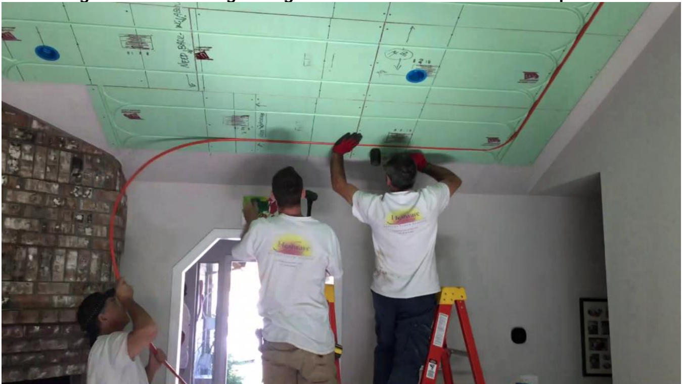
Figure 16 - Installing tubing into the channels of the radiant panels.
