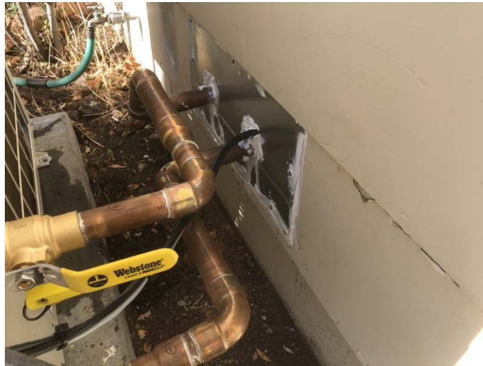
Figure 13: Sealing wall penetrations
