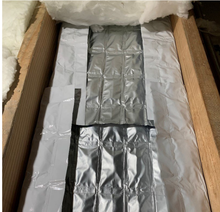
Figure 5. PCM folded or overlapping where necessary. Image credit: Bob Hendron
