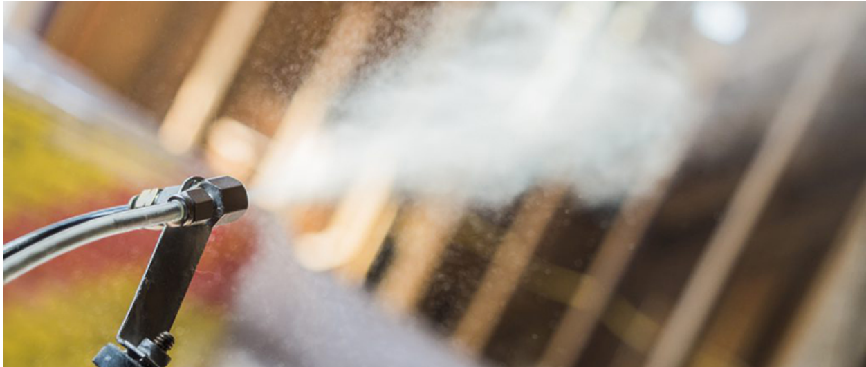
Figure 5: Aerosolized sealant released into the interior of a building.
