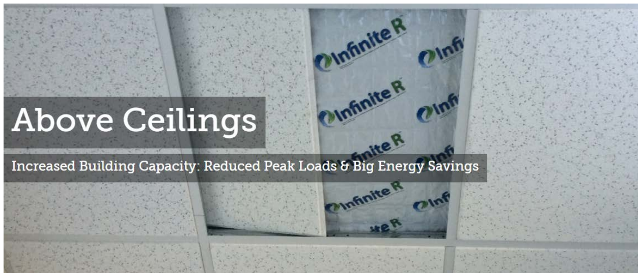
Figure 2: PCM mats installed over a dropped ceiling
